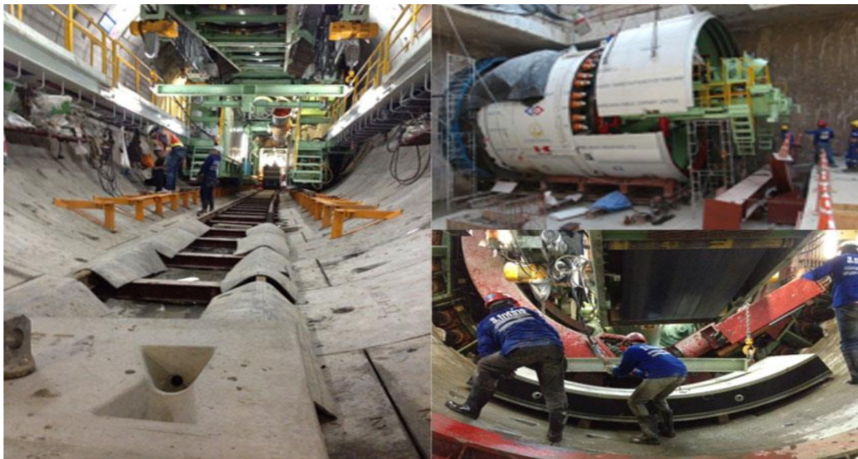
Fig 3. The suway station and tunnel are under constructed.
