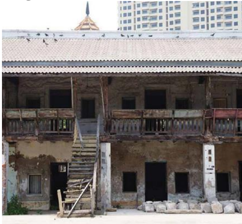
The original warehouse before renovation
