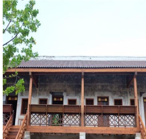
The original warehouse after renovation
